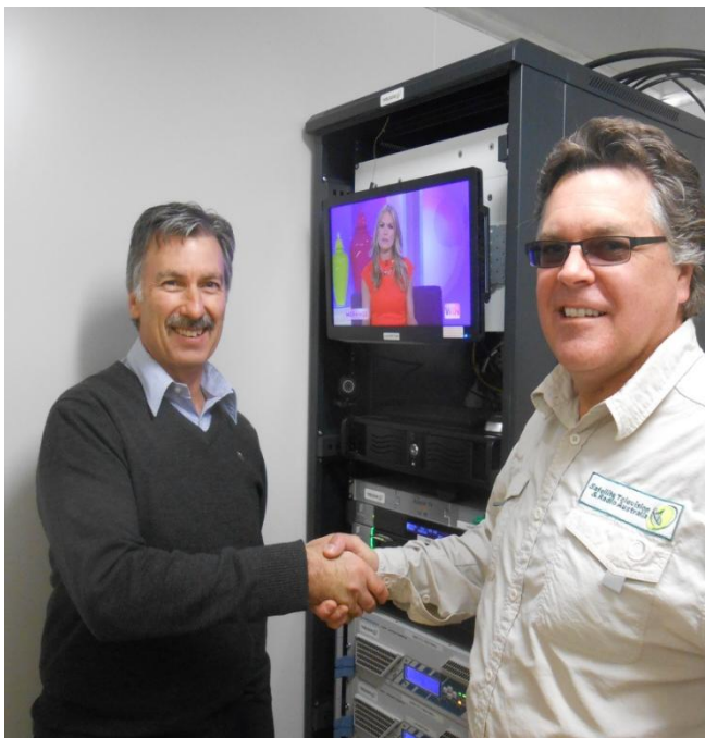
Steven Deckert, Shire of Laverton CEO and Glenn Welsh, General Manager at Satellite Television and Radio Australia inspect the new digital television transmission equipment installed the new communications hut at Hawks Place.
